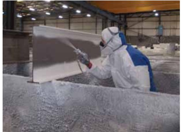
Interchar® 2090 being applied to an I-section
